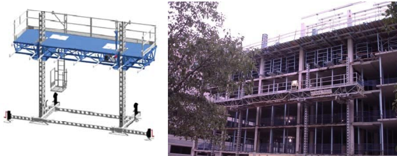
Hydraulic Mast Climbing Scaffold System for Masonry Installation
